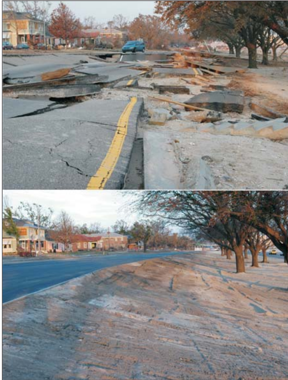
U.S. Highway 90 in Biloxi, Mississippi, before (top) and after repair from damage caused by Hurricane Katrina.
